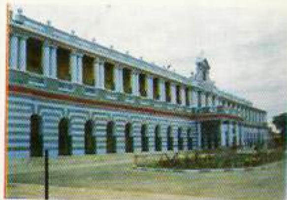
Main Block (View from Left Corner)
