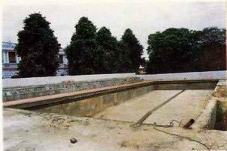
The Swimming Pool (Under construction) 1996
