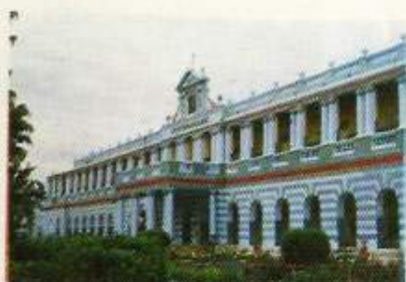
Main Block (View from Right Corner)
