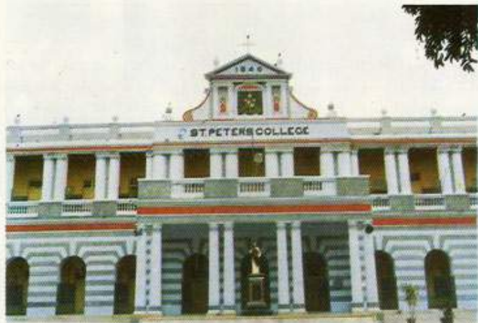
Main Block (Front View) 1846
